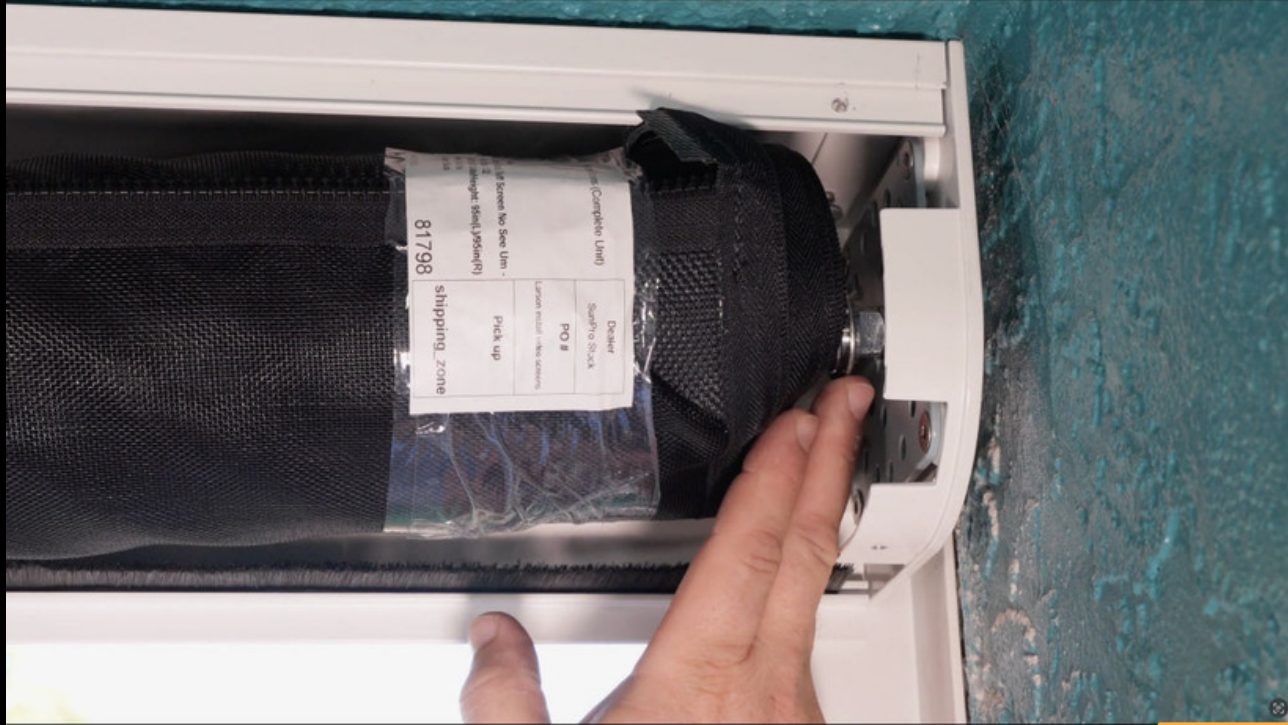
Install and compress roll tube idler end first
